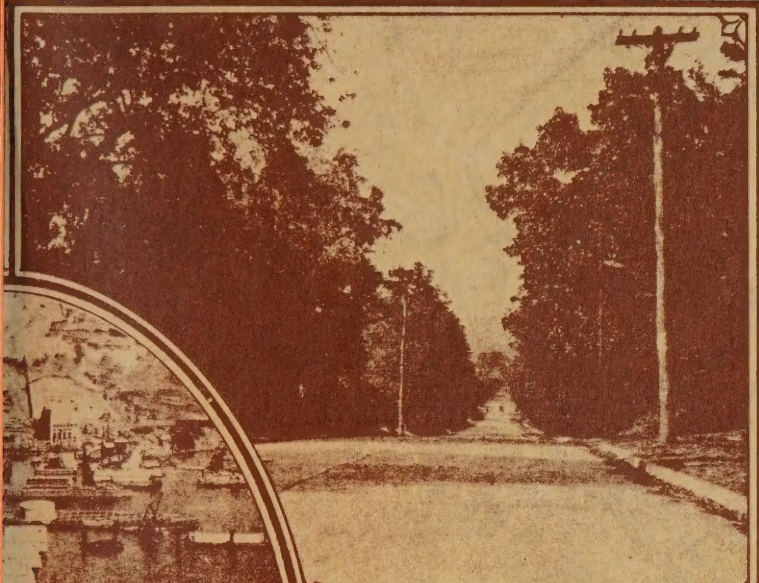
State Highway Route No. 16, Bayard Lane, Princeton, Mercer County
